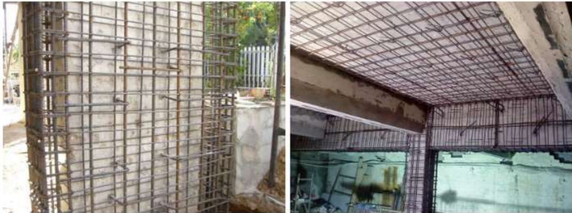
Fig. 3. Seismic upgrading with RC jacketing [Source: Courtesy C. Chrysostomou, TUC].
