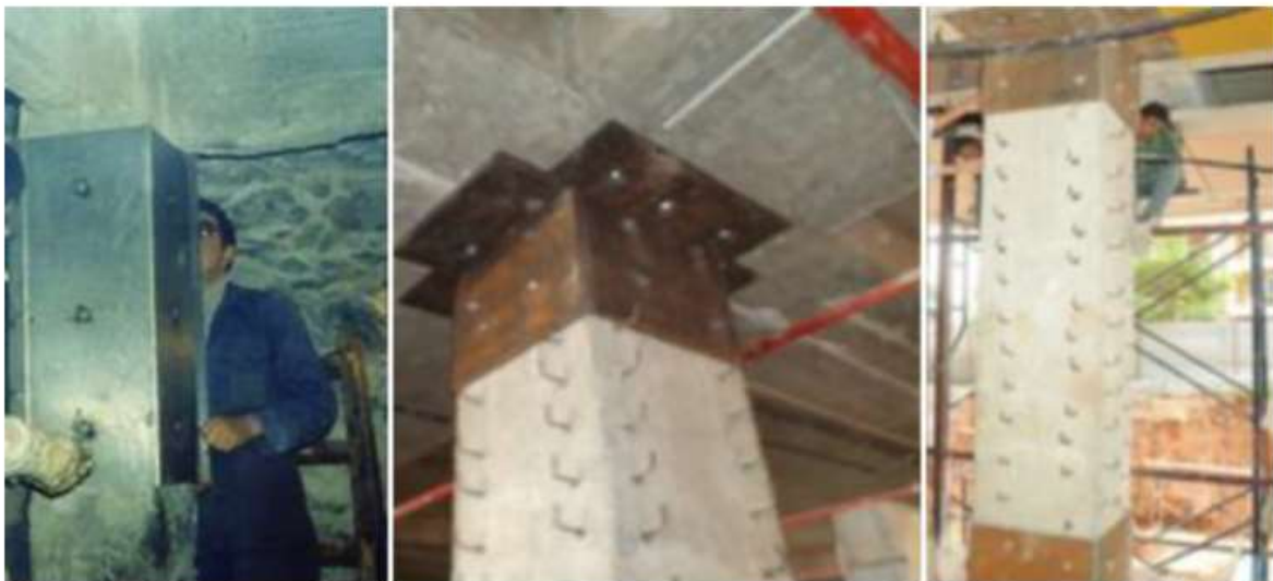
Fig. 4. Seismic upgrading with steel jacketing.
