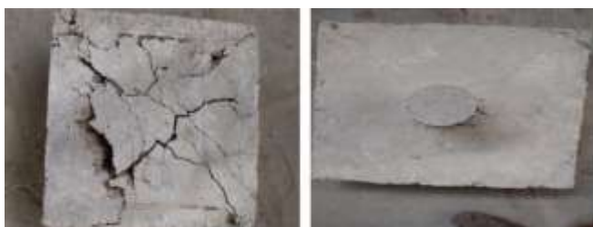
Figure 4.4.1: Typical cracking pattern on the BOTTOM surface of the model slab, cracking pattern on the top Surface of the slab
