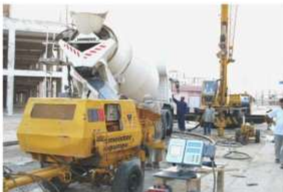
Figure 2: Delivery of cavity filling mix
