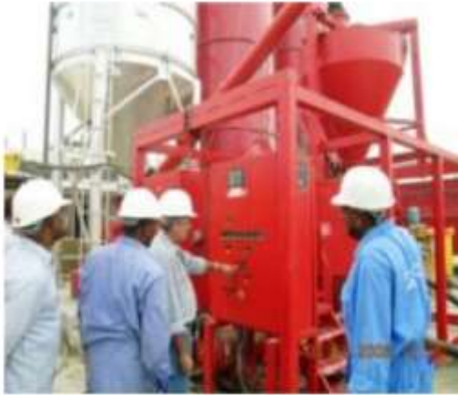
Figure 7: Insite slurry preparation
