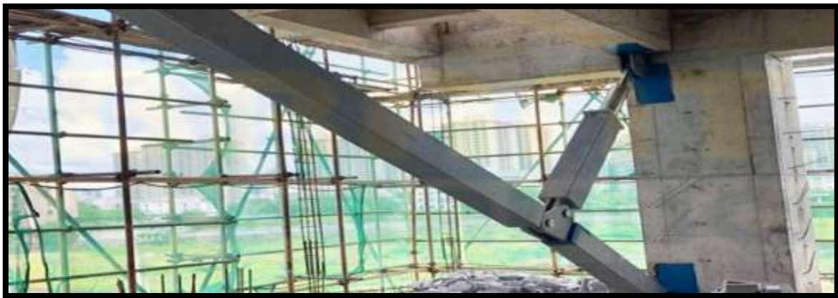
Figure 1.3 FVD fitted in structure
