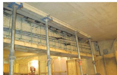
Figure No. 1 External Post Tensioning
