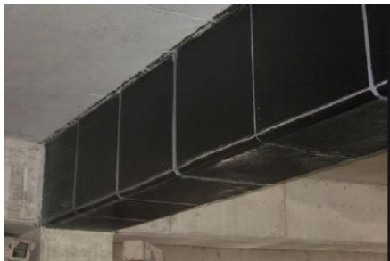
Figure No. 3 Carbon FRP fiber installation
