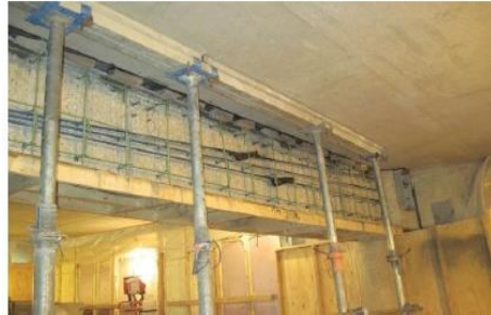
Figure No. 1 External Post Tensioning
